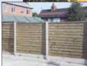
Waneylap Panels with concrete post and base
