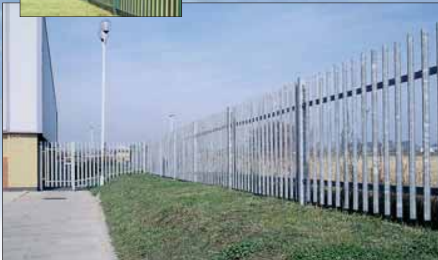
STEEL PALISADE (main picture)
