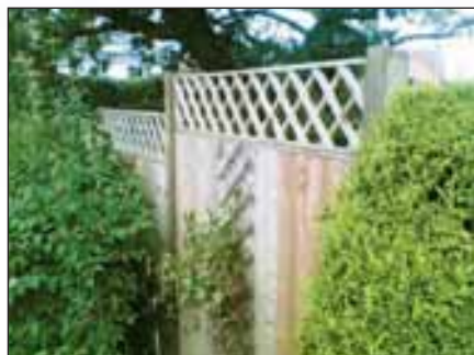
Vertical Board with Standard diamond Trellis
